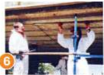
3 Apply MBrace Laminate Adhesive to substrate
