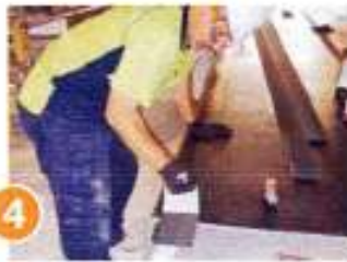
1 Apply MBrace Primer onto prepared concrete substrate
