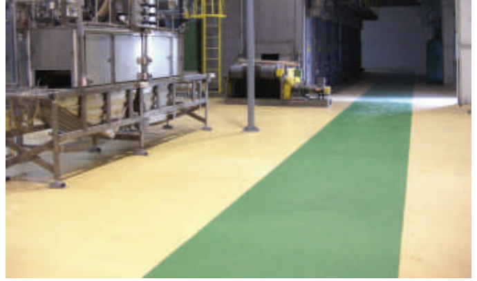
Different colours of UCRETE® DP can be used to delineate walkways and red highlight equipment operating areas.
